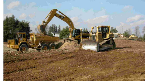
Fire Training Complex
