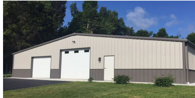
Fire Training Complex- Logistics and Supply
